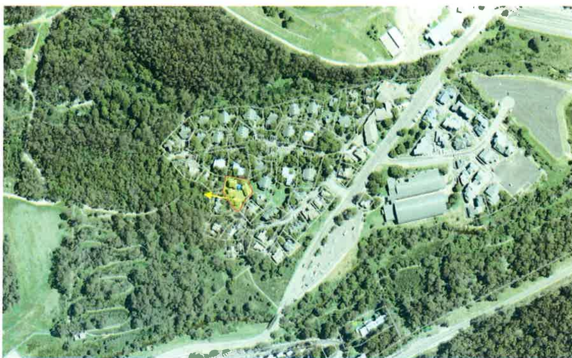
Figure 10: Aerial view demonstrating the location of the vegetation that would have the most influence in the event of a bushfire
